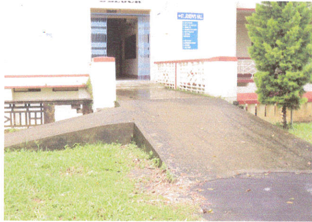
Figure 14: Pedestrian friendly entry to B Block
