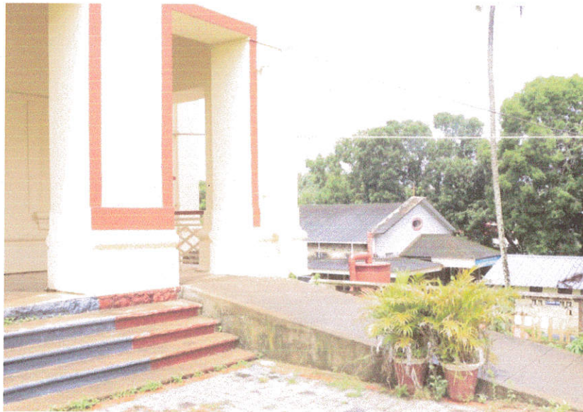
Figure 13: Pedestrian friendly entry to A Block
